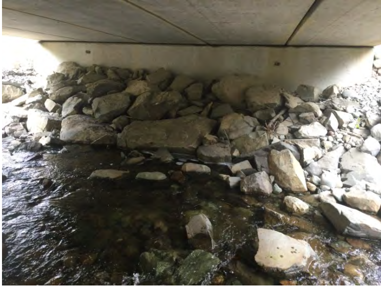
Right Bank Abutment when facing downstream
