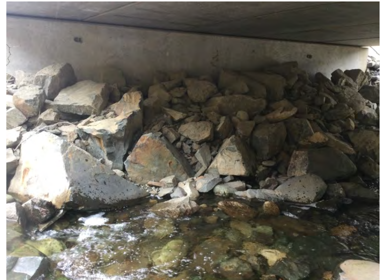
Left Bank Abutment when facing downstream
