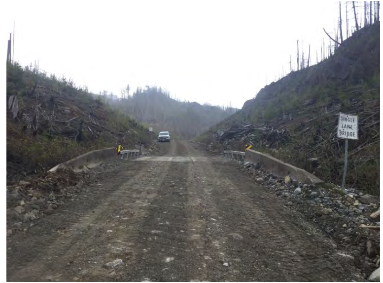
Approach from Right Bank when facing downstream
