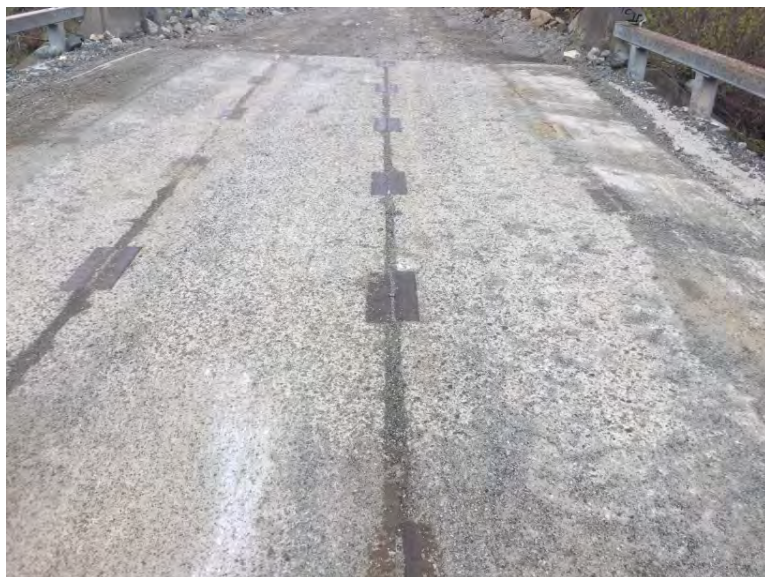
Welded shear connectors
